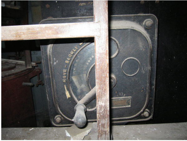
Fig. 9 Detail of the control panel switch, 2009. Image by author. Published with permission from the Government Museum, Chennai.
